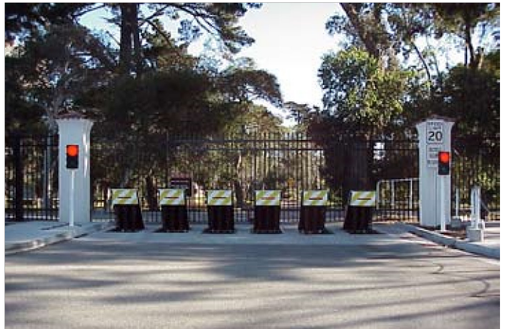
Figure 2: Use of Active and Passive Barriers
